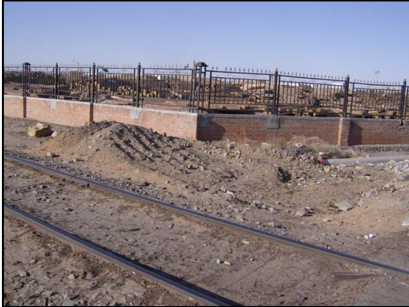
Erlian Port Processing Area for wood
