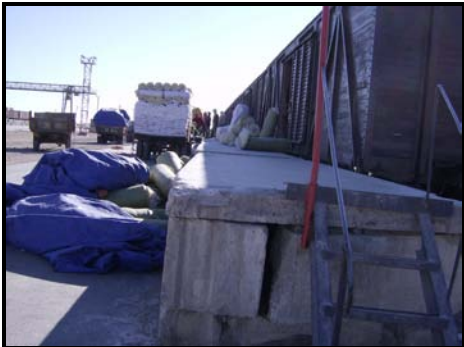
Platform Repairs/Expansion Station #1
